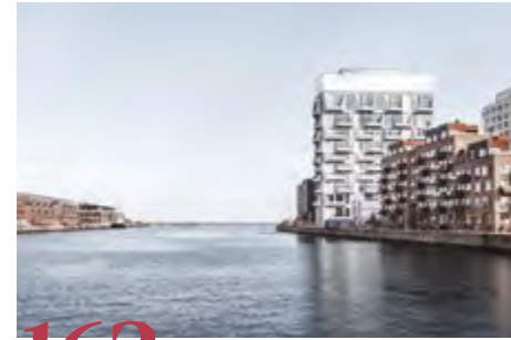
162 SILO IN COPENHAGEN Microtopping®
